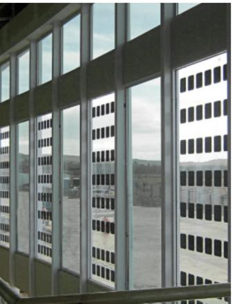
**Curtain walls** are a very popular application for photovoltaic glass in buildings. They allow owners to generate electricity from areas of the building they had never thought of. **Buildings become a real power plant, keeping their design appeal, aesthetics, efficiency and functionality.**
