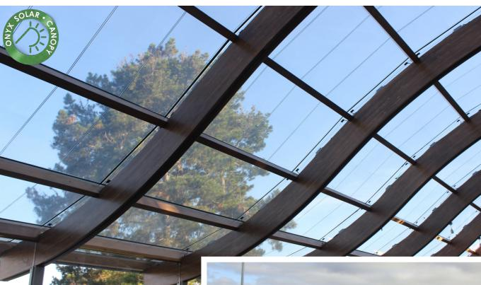
A photovoltaic canopy constitutes a constructive solution which combines energy generation, sun protection and shelter. Depending on the type of canopy, the electricity yielded can be consumed in different ways: self-consumption for surrounding buildings, courtesy lighting, ad. box illumination, back-up systems, and also grid-connection options are available.
